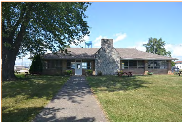
Shelter House (facing north) Estimated Occupancy: 169
