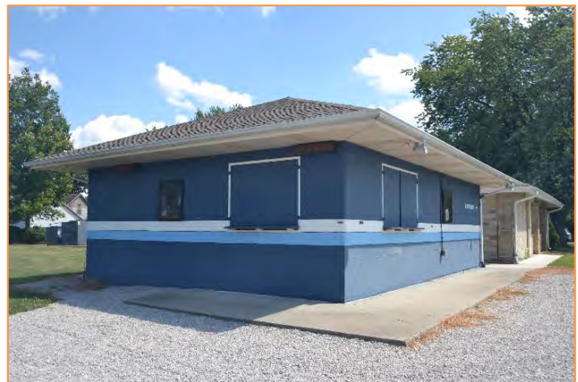
2-Bay Concession Stand / Restrooms (facing southeast)
