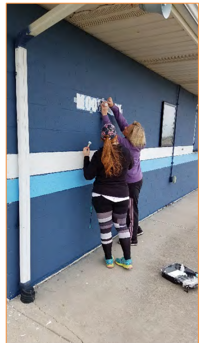
Restroom paint improvements
