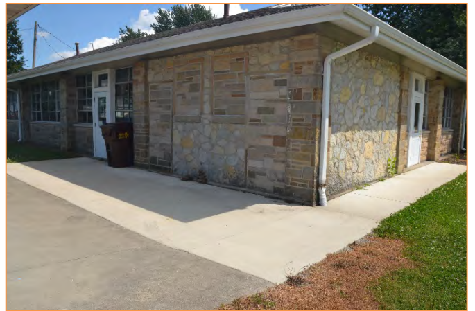
New gutters and soffit at Shelter House
