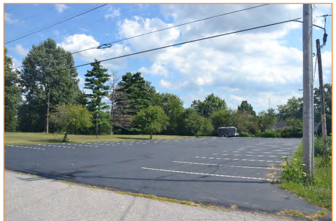
Asphalt parking area (facing southeast)
